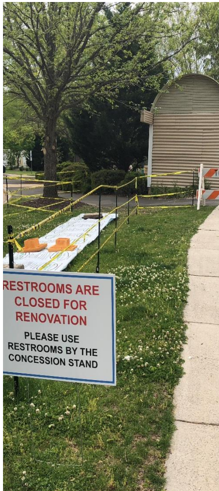
MCP Bathroom Renovation
